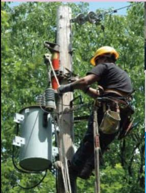
Above: Apprentice Lineman Matt Wiese removes a transformer the "old way," by climbing and using a jib and a block and tackle. This job was part of the tie-line improvement.
